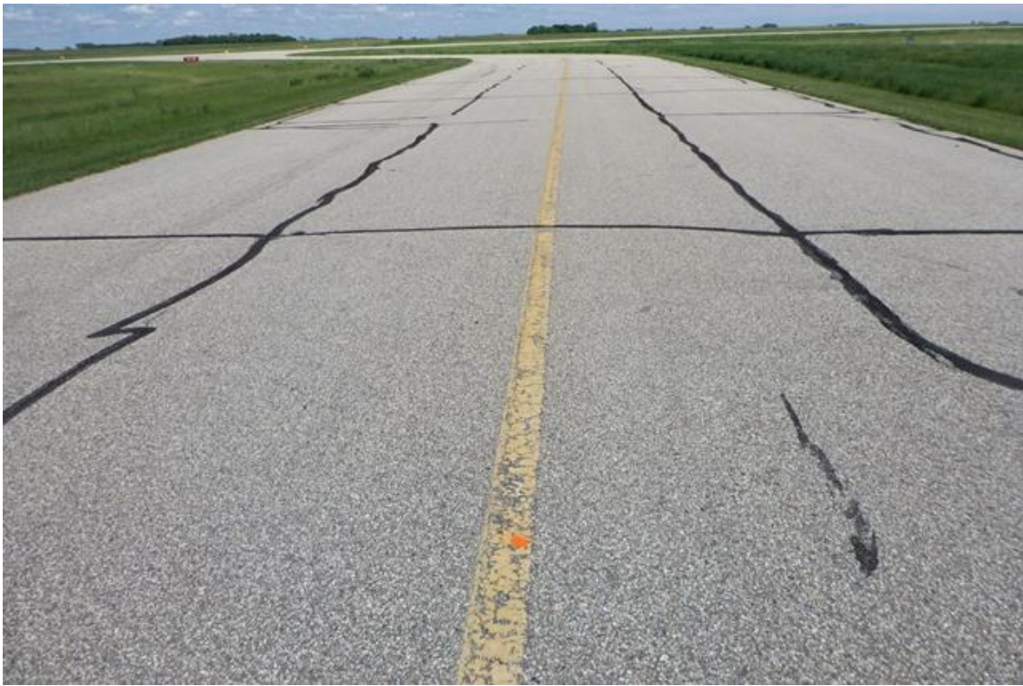
DXX CTA 001 prior to slurry seal (PCI = 63, 6/2/2016)
