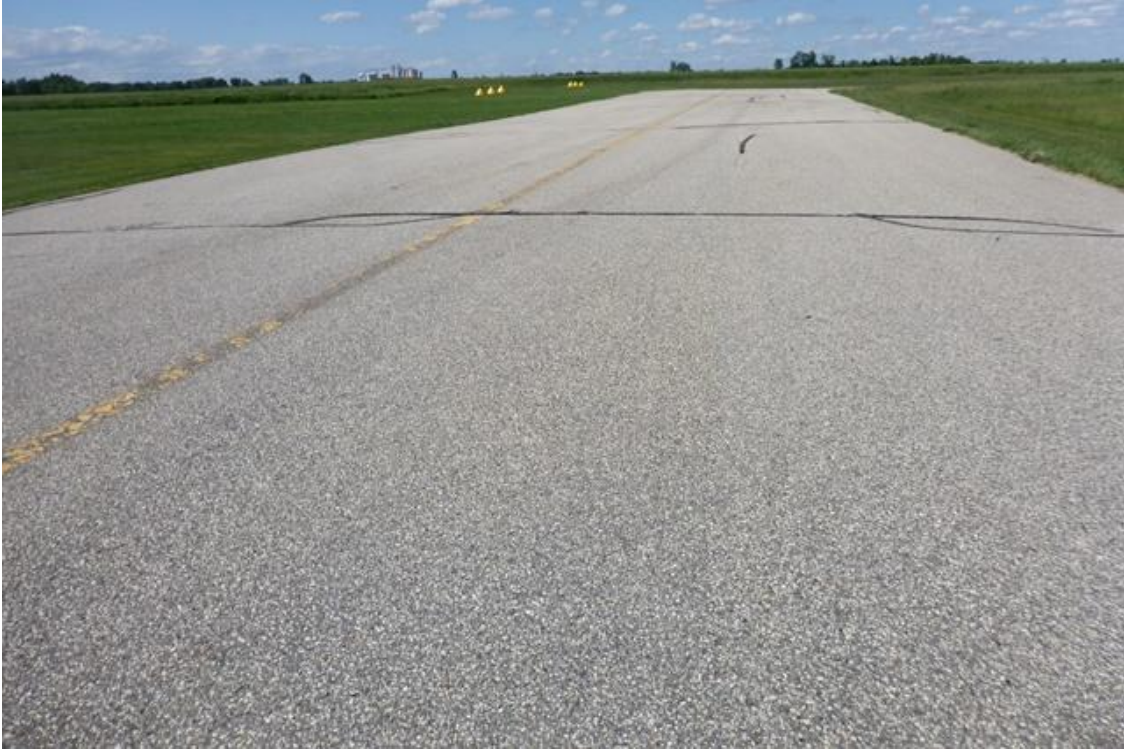
DXX CTB 001 prior to slurry seal (PCI = 60, 6/2/2016)
