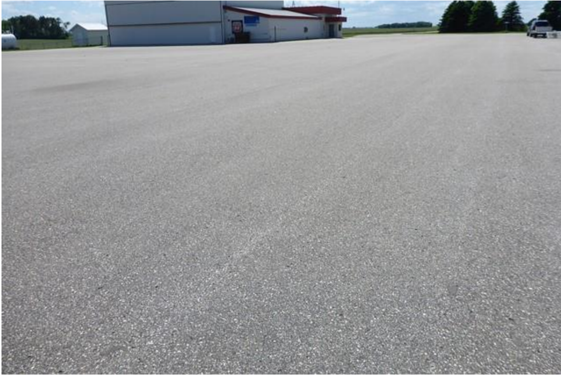
DXX APA 001 prior to slurry seal (PCI = 84, 6/2/2016)
