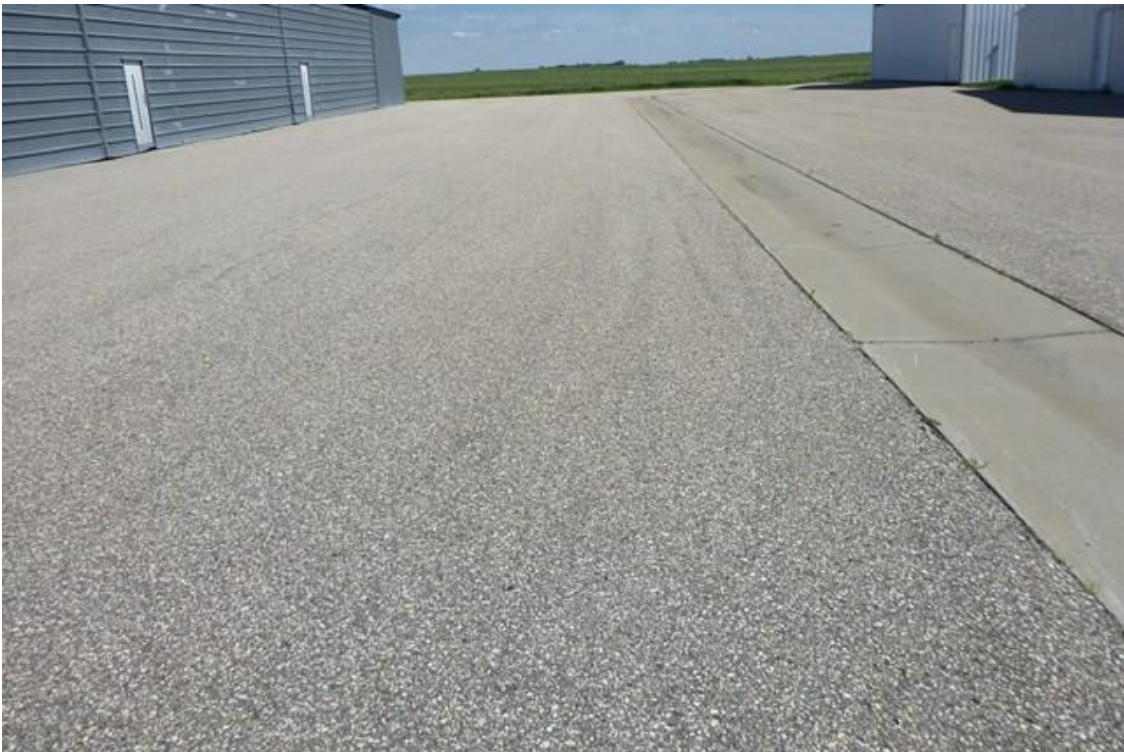
DXX TLA 001 prior to slurry seal (PCI = 73, 6/2/2016)
