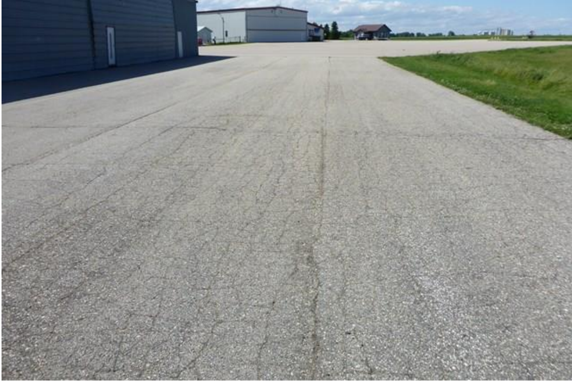
DXX TLA 002 prior to slurry seal (PCI = 17, 6/2/2016)
