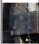
Cap testing can be done in either the vertical or transverse direction. Start at midline near ends or areas of concern.
