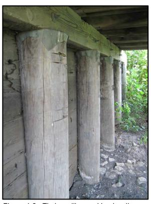
Figure 1.6. Timber piling and backwall forming a timber abutment.
