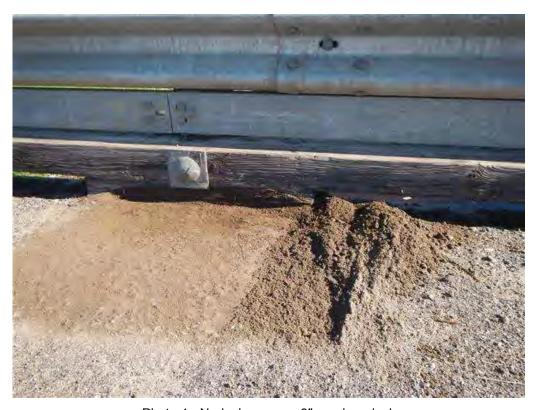
Photo 4 - N. deck-scupper 3" sand on deck
