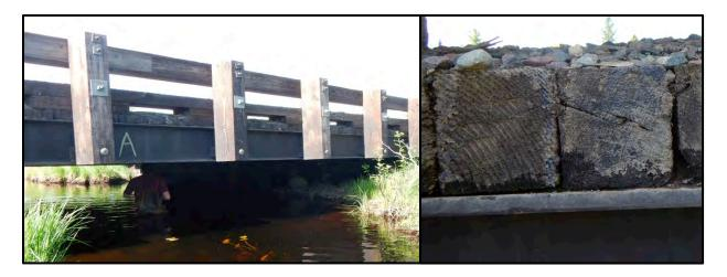
Figure 1.3. Steel beam bridge with a nail laminated timber deck.
