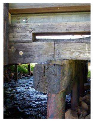
Photo 9 - Pier 2 - South end - Through split continuing 24 inches into cap.
