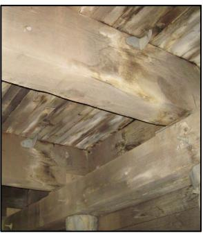
Figure 3.7. Water staining and discoloration caused by water that infiltrated through the bituminous wear layer and nail-laminated deck.
