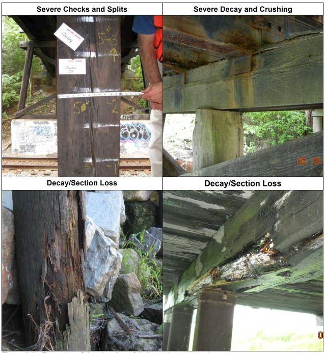
Figure 7.7. Examples of deterioration of timber substructure elements.
