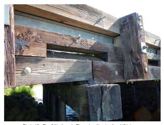
Photo 10 - Pier 2 North end - Through split extending 14" into cap.
