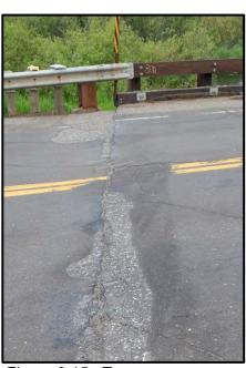
Figure 3.15. Transverse cracking that occurs over the beginning of bridge abutment.
