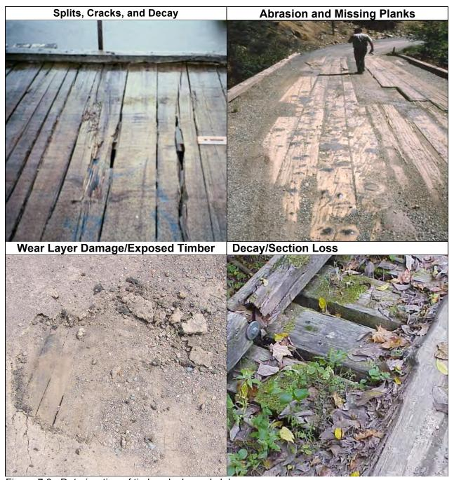
Figure 7.3. Deterioration of timber decks and slabs.
