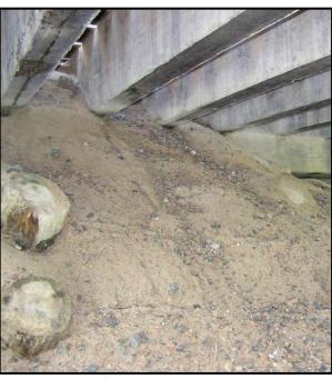
Figure 3.22. Sand and gravel are covering the timber abutment cap and the longitudinal timber beams, holding moisture against these elements.
