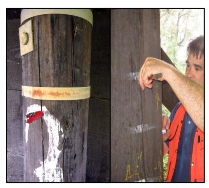
Figure 4.3. Probes are used to assess the depth of cracks, checks and through splits in timber bridge elements.
