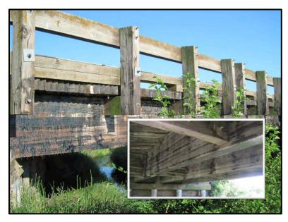
Figure 1.2 Glulam beam timber bridge construction.
