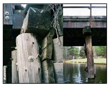
Figure 3.20. Rotation of timber pilings and pile caps in an abutment (left) and timber pier (right).
