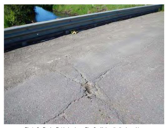
Photo 2 - Deck - Pot hole above Pier 2 with longitudinal cracking
