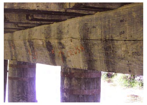
Figure 3.13. A long horizontal split provides an opportunity for moisture passing through the timber deck to enter the abutment cap, leading to substantial decay.
