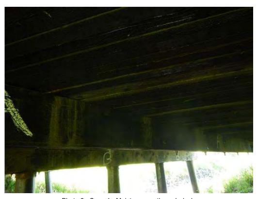
Photo 8 - Span 1 - Moisture pen. through deck.
