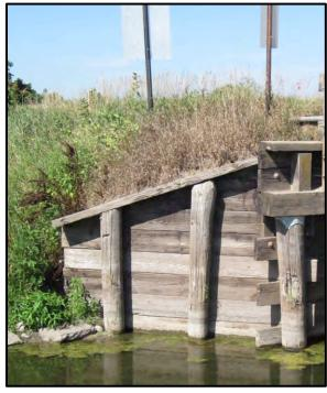
Figure 1.8. Timber piling, piling and cap board forming a timber wingwall.
