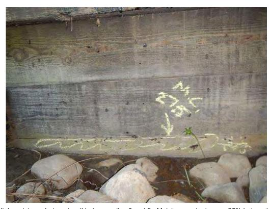
Photo 12 - High moisture abutment wall between piles 8 and 9. Moisture content over >25% but no decay present.
