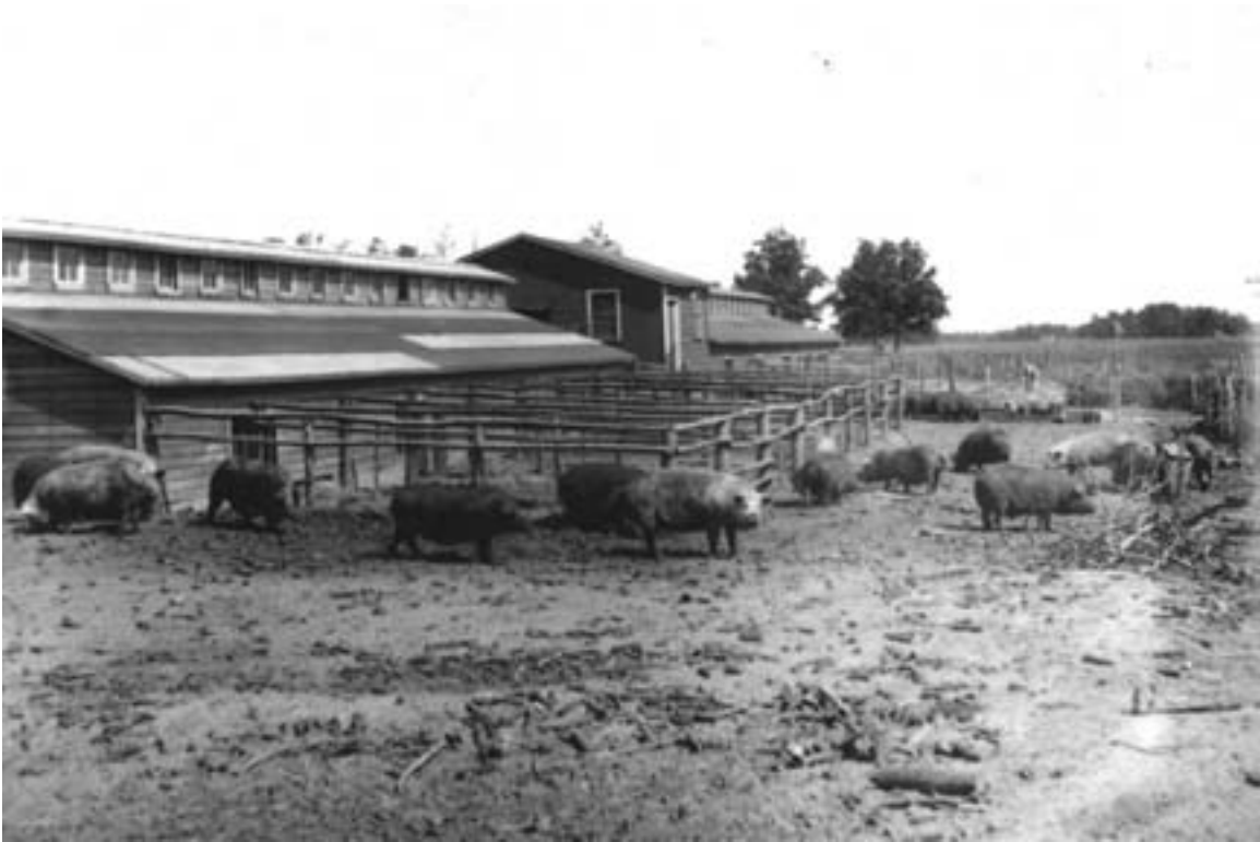
Permanent hog barns of this design were built in Minnesota by the 1890s. The position of the windows indicates that the house had two rows of pens – one lit by the south-facing first-story windows and the other by windows at the clerestory level. By the 1920s disease prevention programs were discouraging farmers from using dirt-surfaced hog yards like this one. Location unknown, 1913. (MHS photo)
