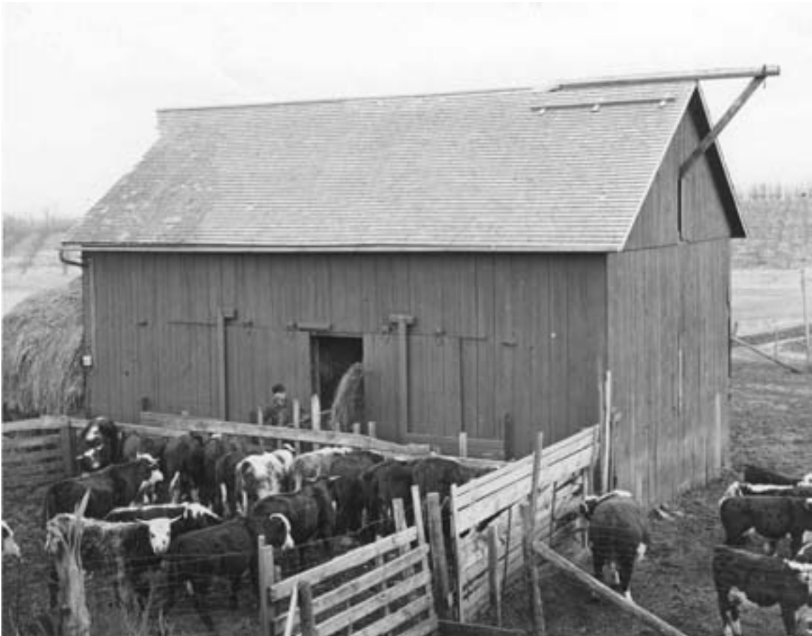
A fully-enclosed hay barn, photographed in 1932, that had typical sliding doors in the side wall, a brace and pulley on one end, and a hay hood on the other end. The photo shows additional hay stacked outside. It is interesting that the barn had electric wires leading to it. Benitt Farm, location unknown, 1932. (MHS photo by Nasvik)
