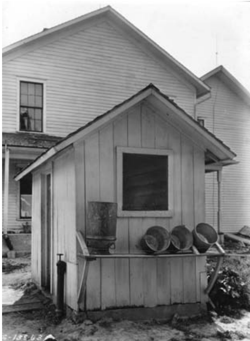
An adequate milk house could be as small as 8' x 8', although a 10' x 12' design was more accommodating. This house had a concrete foundation, wood siding, and an outside drying rack, all typical. The black device (with handle) near the door was probably an insulated water shut-off valve. Believed to be Douglas County, circa 1950. (MHS photo)
