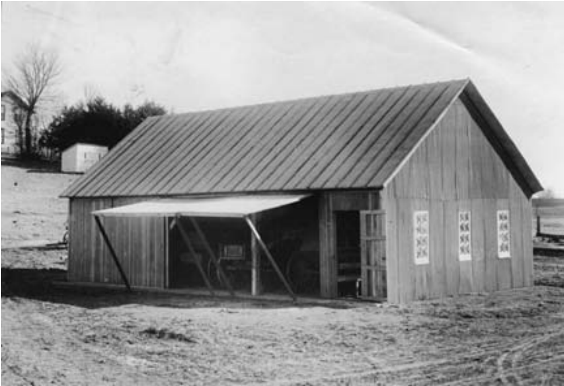
An implement or machine shed. It had a standing seam metal roof and the walls were sheathed in corrugated metal. Location unknown, circa 1910. (MHS photo by Harry Darius Ayer)
