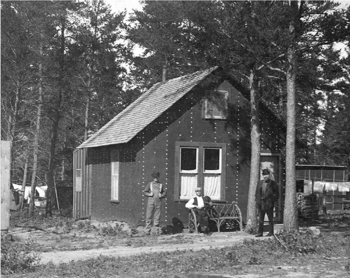
A farmhouse and outbuilding covered with tar paper, a common sheathing material that was inexpensive and readily available. The paper easily came loose with conventional nails, so it was secured with wide-headed tacks or strips of lath. It lasted longer in wooded areas where the trees offered some protection from the wind. Asphalt roofing material, available in shingles or rolls, was a more durable alternative. Cass County, circa 1910. (MHS photo)
