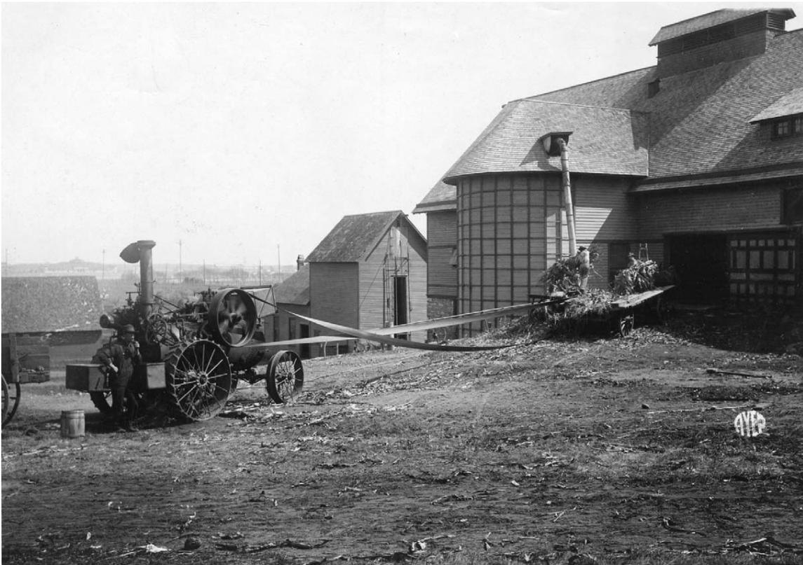
The development of silo loading equipment encouraged silo construction. Pictured above, men chop bundles of cornstalks and blow them into a silo. The chopping and blowing equipment was powered via a belt from a steam traction engine or "tractor". The silo was built of horizontal wood and was incorporated into the massing of the barn. Location unknown, circa 1910. (MHS photo by Harry Darius Ayer)
