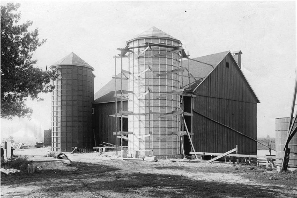
Some horizontal wooden silos were reinforced with vertical boards and then a set of iron bands. This silo, which had both vertical boards and bands, was under construction. Blackinere Farm near Albert Lea, circa 1910. (MHS photo by Harry Darius Ayer)
