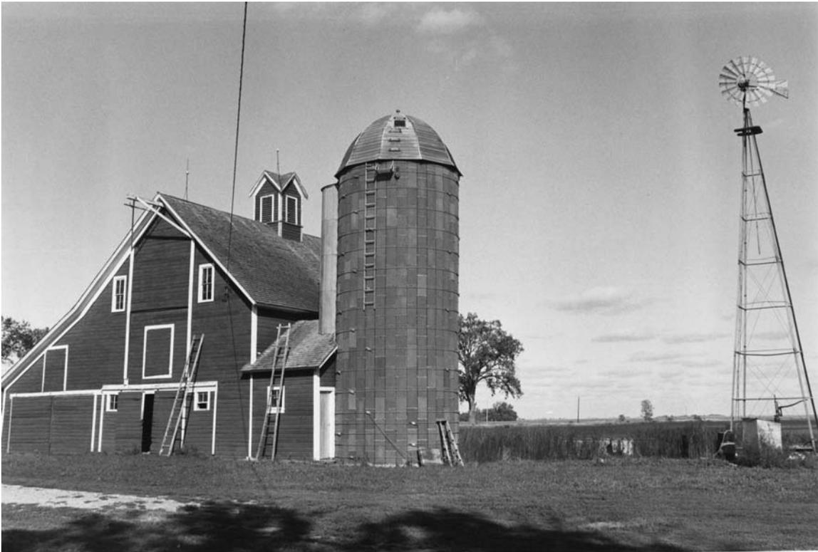
Cement stave silos were introduced in 1905. The staves were assembled either dry or with mortar. The silo interior was usually plastered with a thin layer of concrete to make it waterproof. Most cement stave silos had reinforcing hoops, which could be either flat bands or round rods. In the mid-20th century, cement stave silos were probably the most common type of silo being built in Minnesota. Elfstrom Farm, Traverse County, 1983. (MHS photo)
