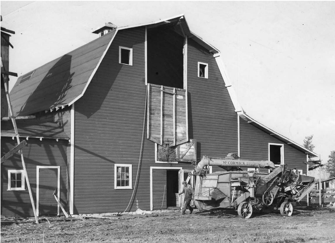
Farm building design responded to mechanization. Threshing machines made three-bay threshing barns obsolete. Mechanized hay carriers and hay forks allowed farmers to handle more hay, and hay lofts – like this barn’s upper story – grew larger. Threshing machines, like the one shown here, and their large crews were replaced beginning in the mid-1930s by relatively small, tractor-pulled combines that individual farmers could afford to own. Koochiching County, circa 1935. (MHS photo by Russell Lee)
