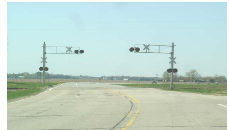
(Photo looking west): Existing Highway 14 at-grade crossing of the DM&E Railroad, which is located east of Highway 218.
