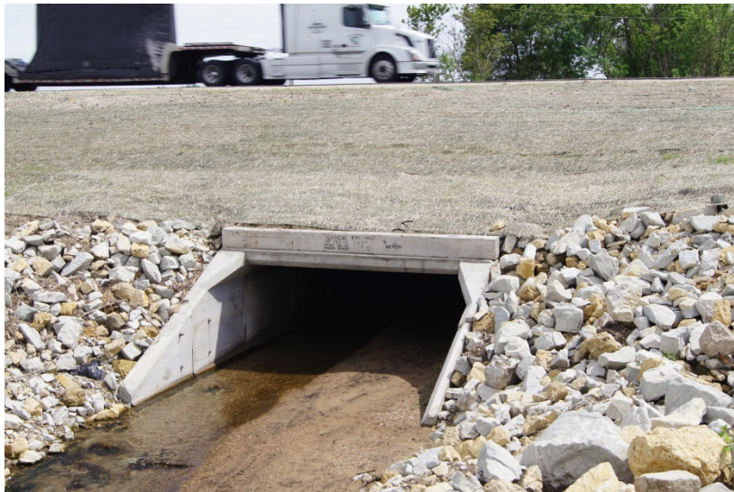
Figure 20 - Culvert Headwall
