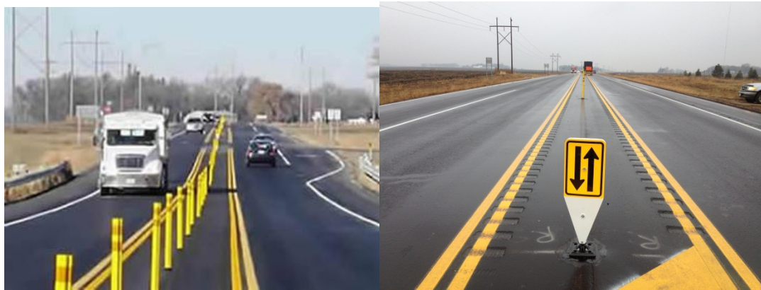
Figure 13 – Center Buffer Zone with Delineators (USTH 14 west of Mankato)
