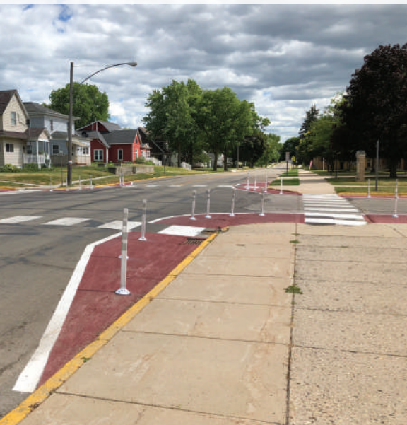
Hwy 22/3rd St temporary curb extension
