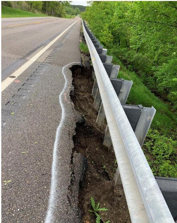
Figure 6. Washout Area at the Guardrail
