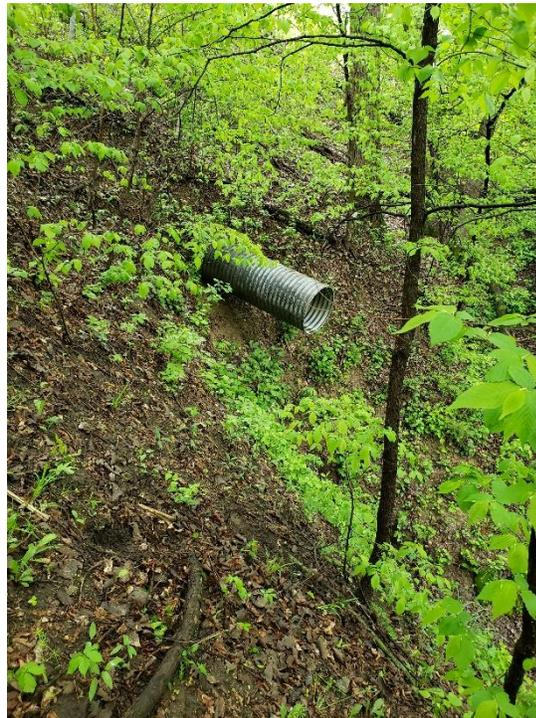
Figure 7. Erosion at the Culvert End
