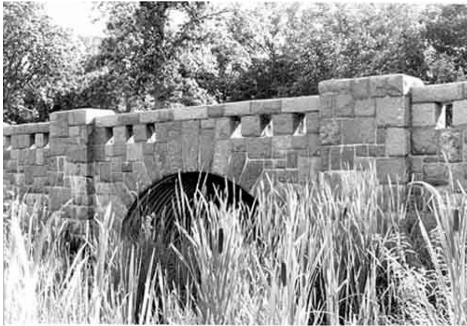
Fig. 20. Garrison Pedestrian Underpass (Bridge 5265), Aug. 1997.
