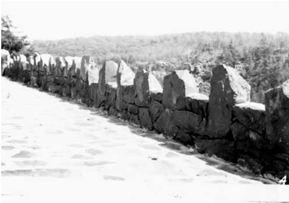
Fig. 46. Taylors Falls Overlook - South, July 1937 (Mn/DOT photo).
