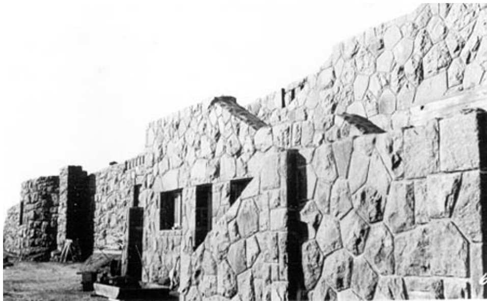
Fig. 21. Gooseberry Falls Concourse, Dec. 1939 (Mn/DOT photo).
