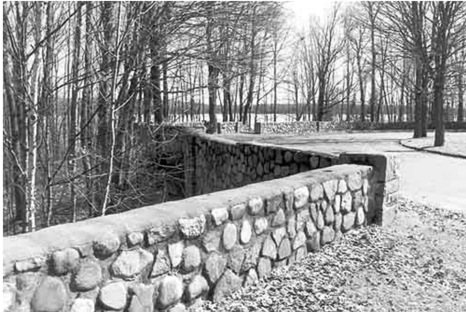
Fig. 55. Willow Lake Roadside Parking Area, Aug. 1997.
