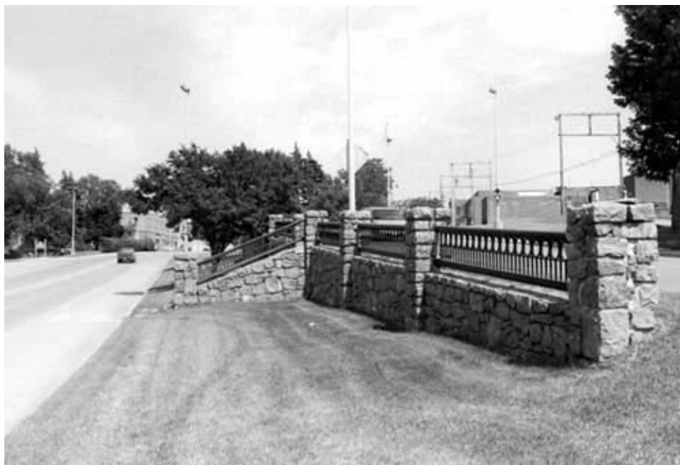
Fig. 38. Redwood Falls Retaining Wall, Sept. 1997.
