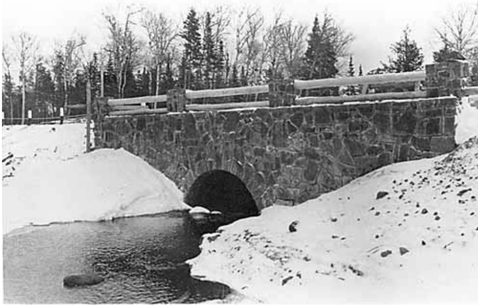
Fig. 44. Spruce Creek Culvert (Bridge 8292), Circa 1935 (Mn/DOT photo).
