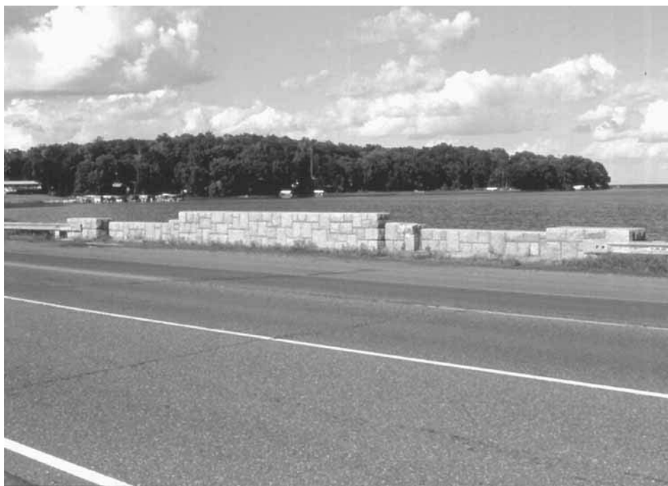
Fig. 54. Whitefish Creek Bridge (Bridge 3355), Aug. 1997.
