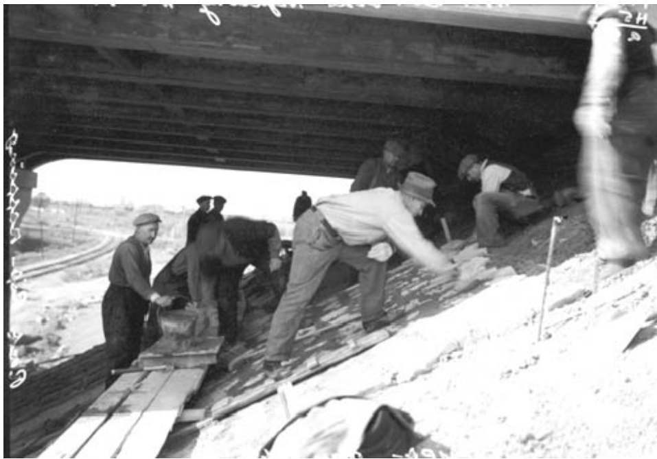
Fig. 4. WPA workers installing rock riprapping under Bridge 5399 on T.H. 100 in Golden Valley, 1936 (MHS photo).
