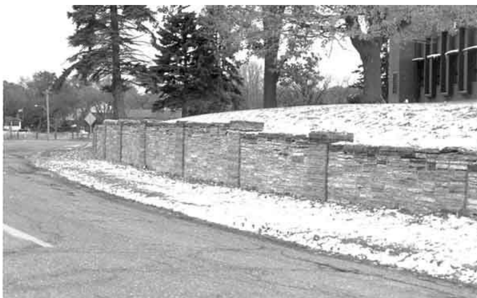
Fig. 50. TH 100 at TH 55 Retaining Walls, Nov. 1997.
