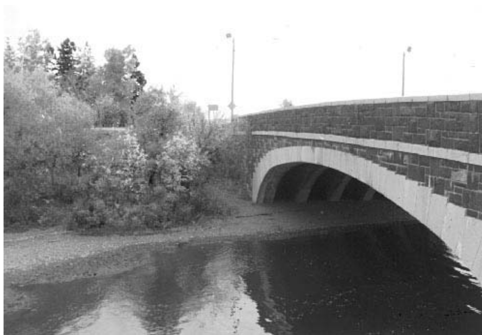
Fig. 29. Lester River Bridge (Bridge 5772), Oct. 1997.
