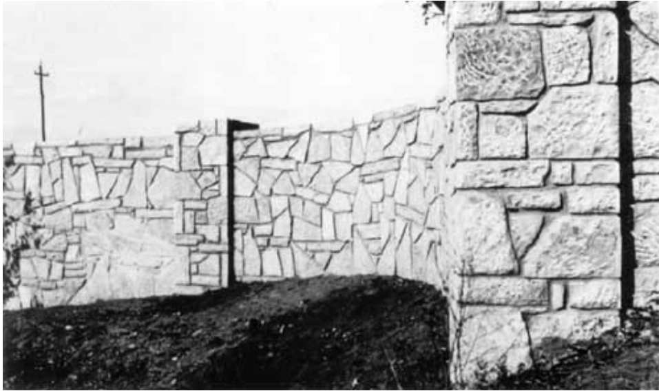
Fig. 36. Preston Overlook, Nov. 1937 (Mn/DOT photo).
