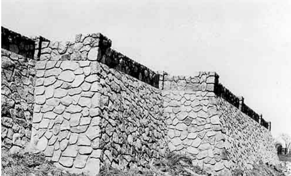
Fig. 18. Garrison Concourse, May 1937 (Mn/DOT photo).
