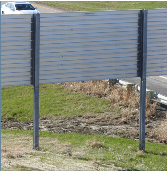
Figure 3.4: I Beam Sign with Extruded Aluminum Panels
